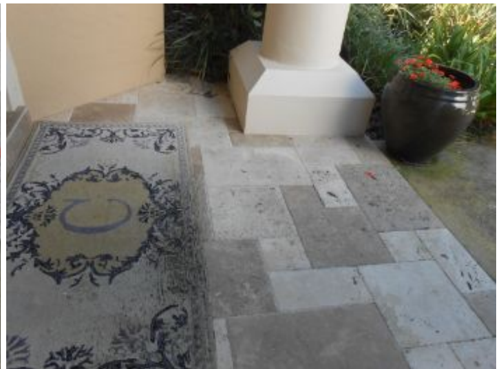
Tiled Entry way
