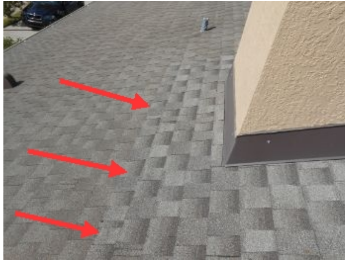
repaired area at chimney
