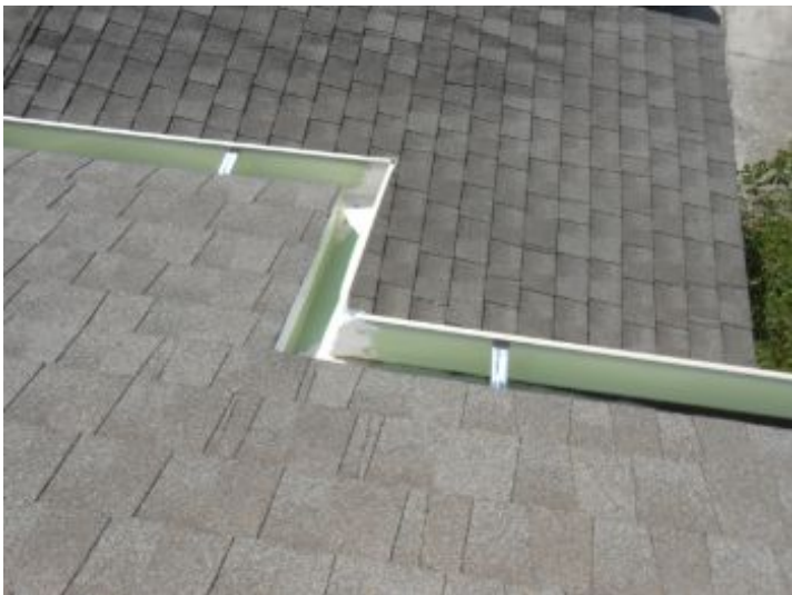
No Concerns with gutters
