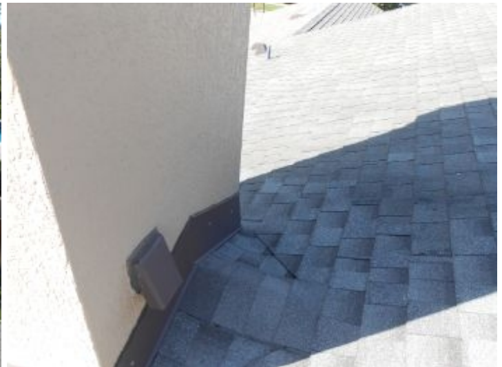
Repaired area at chimney (cricket installed)
